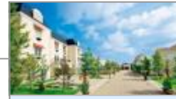
Canalside La La Chance
