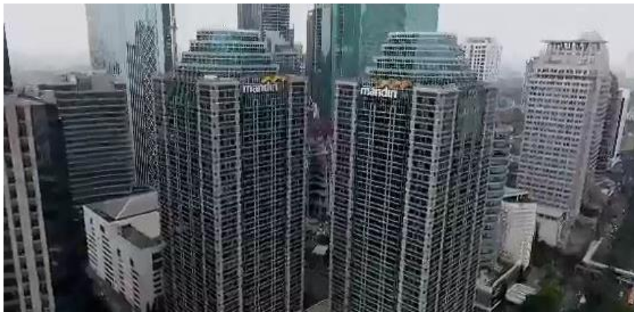
The company occupies the 9 th and 10 th floors of the Menara Mandiri building
